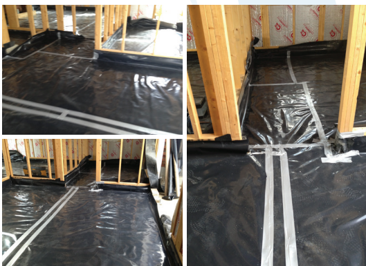
FIGURE 3: Taping membrane
