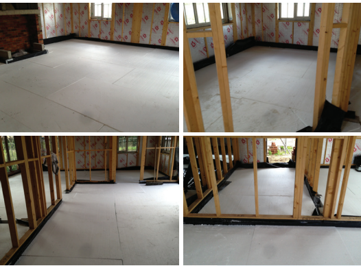
FIGURE 4: Fitting insulation
