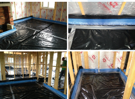
FIGURE 6: Fitting Perimeter Expansion Joint
