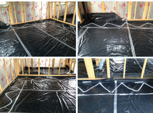
FIGURE 5: 500 gauge slip membrane installation
