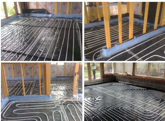
FIGURE 7: Fitting underfloor heating pipe work
